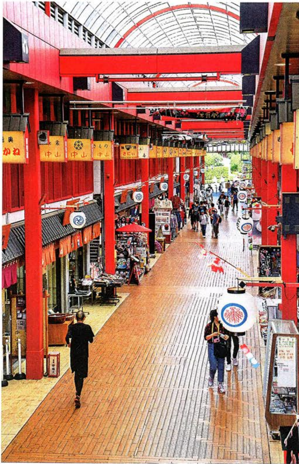
Asakusa Temple / West entrance renewal
