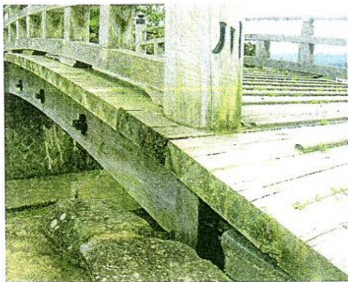
Construction Before use
