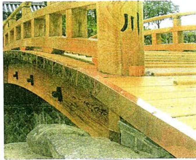
After construction use
